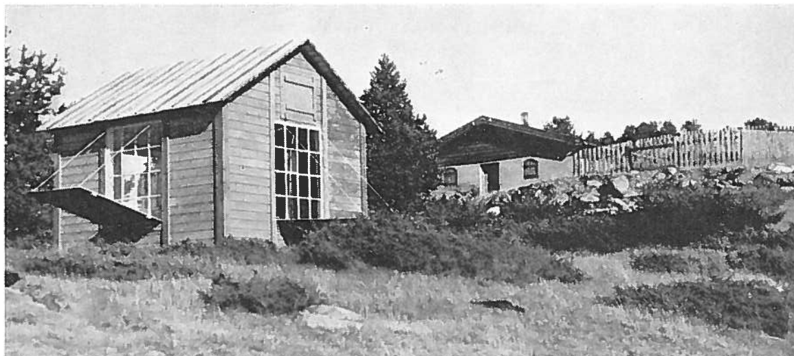
Fig. 11. View to the north-east; absolute house in foreground, variometer house in background. (Photo G. G., June 1955).
