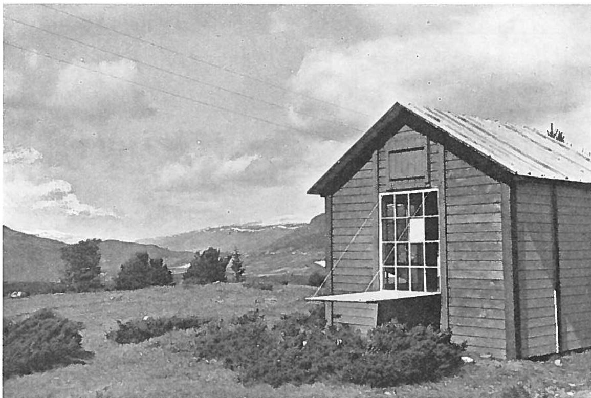
Fig. 4. View to the north-west; absolute house. (Photo G. G., June 1955).
