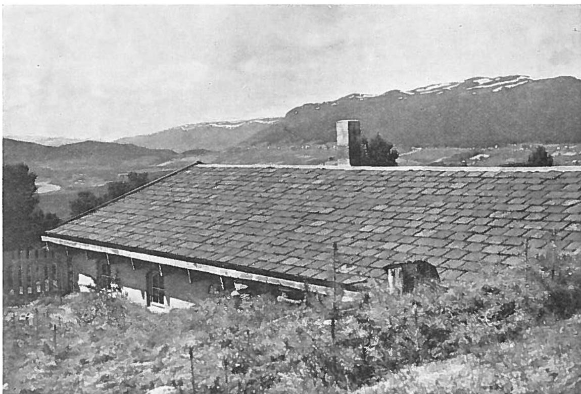
Fig. 5. View to the north-west; variometer house. (Photo G. G., June 1955).
